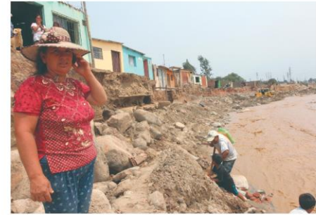
Flood victim on the east side of Lima views her home as a flash flood scoured the bank, causing houses to collapse. (Photo by Andrew Huxton)
